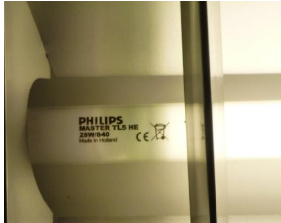
Lamp wattage clearly visible
