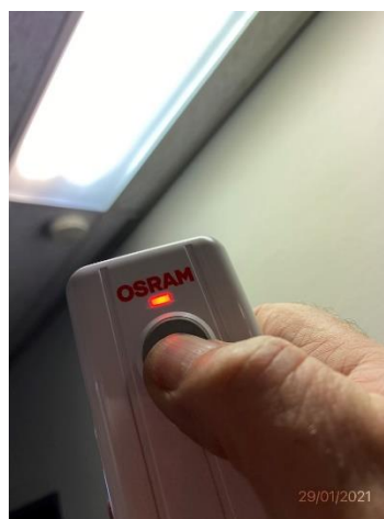
Figure 23: Photograph showing ballast discriminator test
