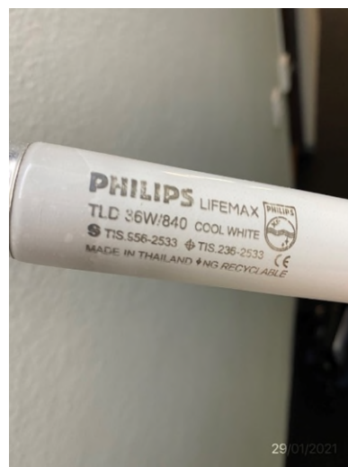
Figure 19: Photographs showing 2x36W T8 fluorescent tubes.
