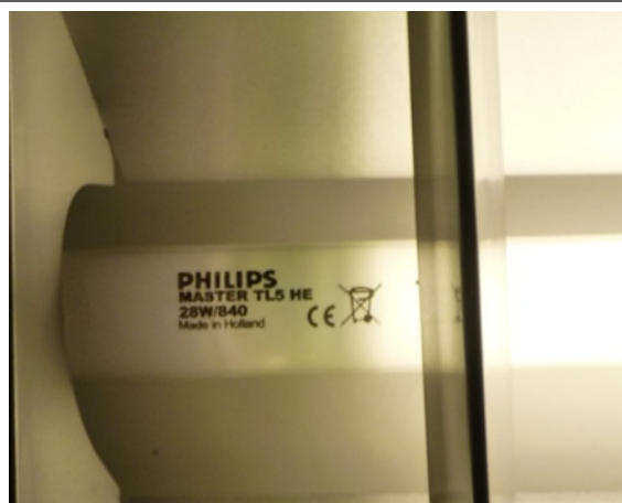
Lamp wattage clearly visible
