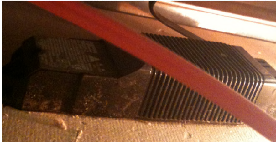
Figure 5: Magnetic transformer in ceiling space
