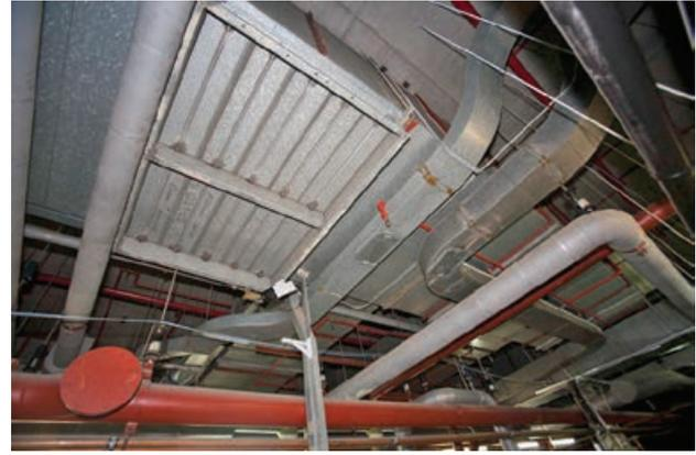
**Air plenum of an air handling unit showing motorised outdoor air and return air volume control dampers**
