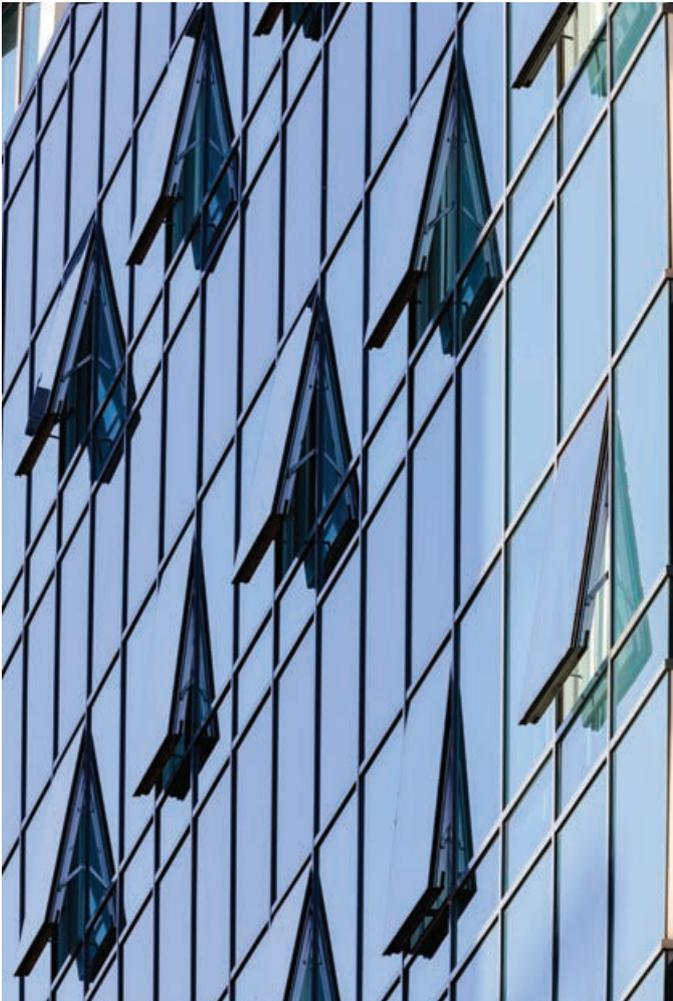
**Night purge aims to reduce the use of mechanical cooling in buildings by flushing the building with cool outdoor air using natural ventilation at night**
