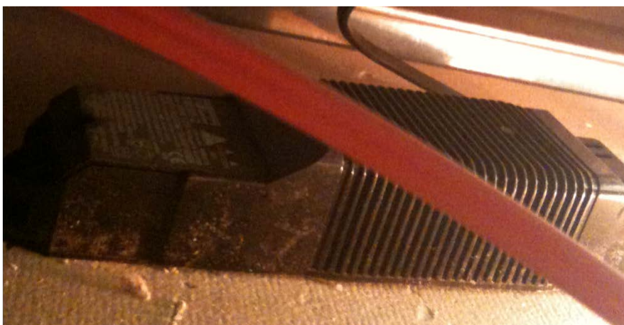
Figure 5: Magnetic transformer in ceiling space
